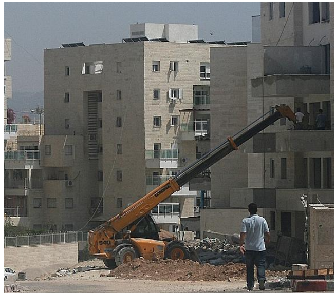
Modi'in Ilit – (near Ramallah) – Apartment buildings in final stage of construction. August 2010 – Al-Haq©
