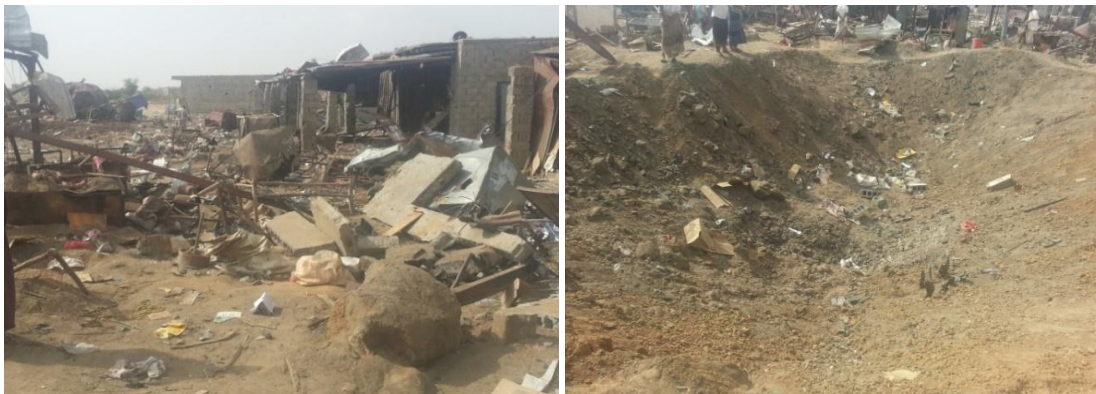
Figure II Damage to the Khamees market
