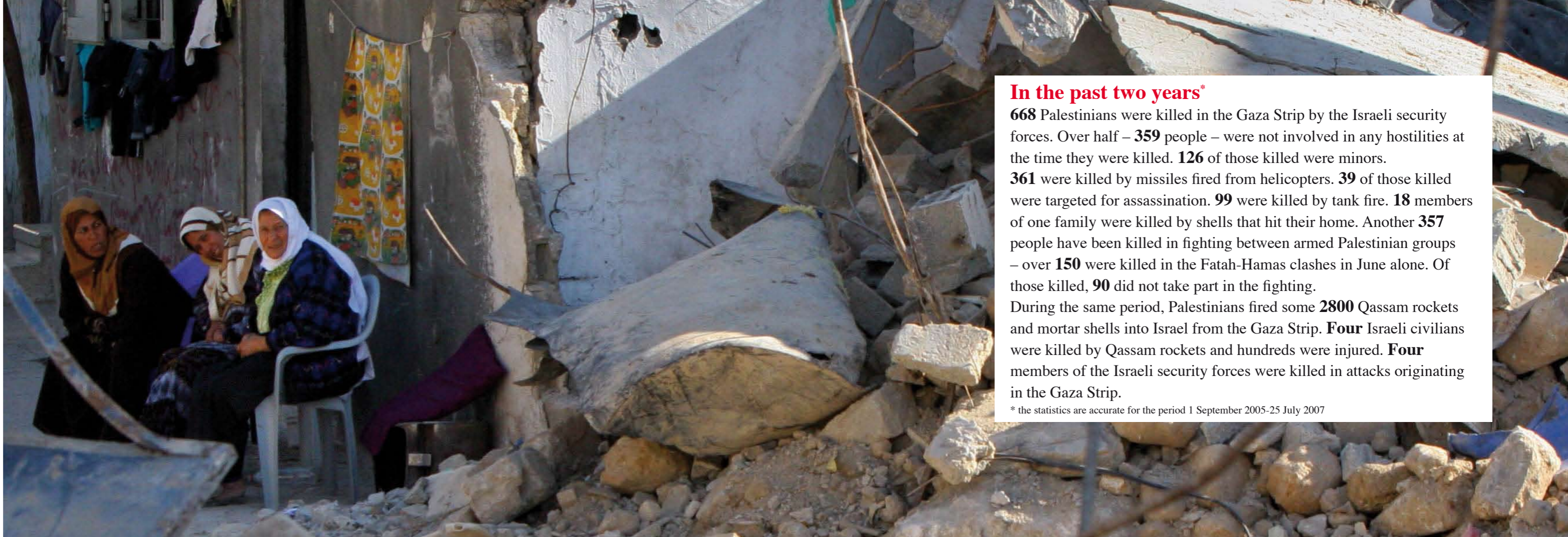
Palestinian family beside house demolished in military operation in Beit Hanoun. Photo: Khalil Hamra, AP
